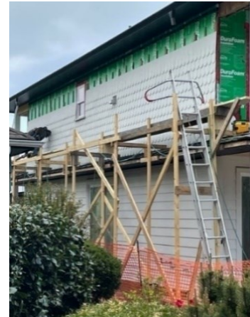
White siding being installed over the green layer of exterior insulation.
